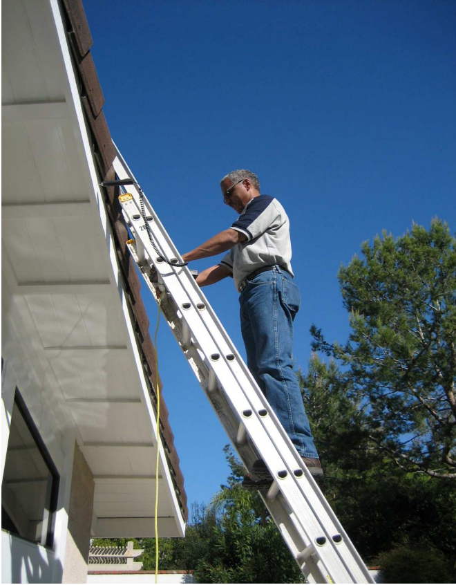
Figure 5. A high-degree of difficulty local-treatment; inspection and treatment conducted in Lake Forest, CA. Included in image is V. Lewis, UC Berkeley.
