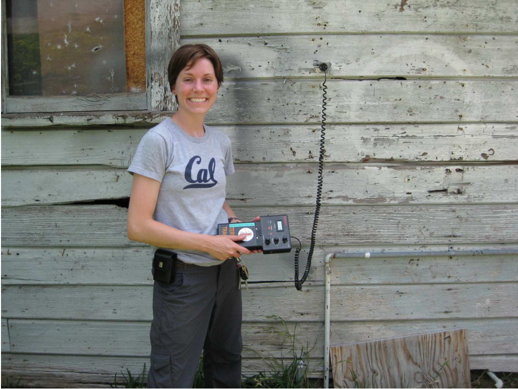
Figure 2. AE monitoring of board for drywood termite activity in Glendora, CA. Include in image is R. Tabuchi, UC Berkeley.
